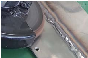
Removing blue weld discoloration
