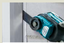
Cutting window putty, silicone
