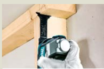
Wood flush cutting
