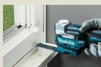
Removal of window frame
