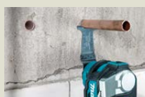
Copper pie flush cutting
