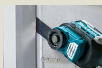
Cutting window putty, silicone
