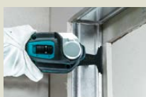
Door opening work
