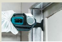
Door opening work
