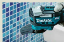
Routing joints on wall tiles
