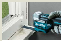
Removal of window frame
