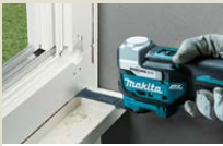
Removal of window frame
