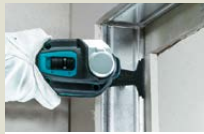
Door opening work
