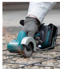
Cutting- Masonry & Concrete
