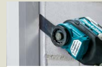
Cutting window putty, silicone
