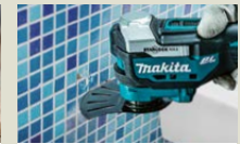
Routing joints on wall tiles
