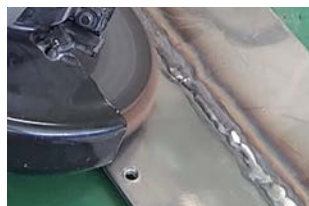
Removing blue weld discoloration
