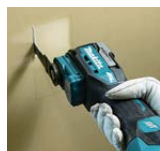
Cutting plasterboards
