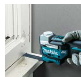
Removal of window frame
