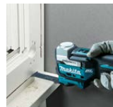
Removal of window frame
