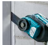
Cutting window putty, silicone
