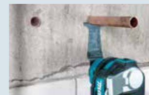
Copper pipe flush cutting
