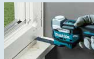
Removal of window frame
